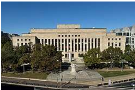
Federal courthouse in Washington, D.C.
